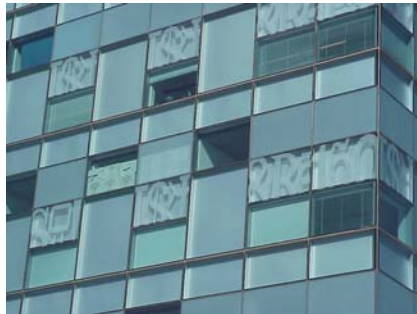
ASU Communications Building All-glass aluminum curtainwall WWR approximately 15%
