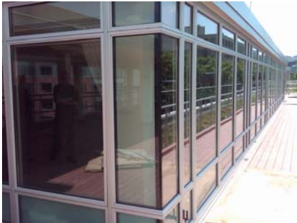
UPenn English House Operable aluminum windows WWR approximately 80%
